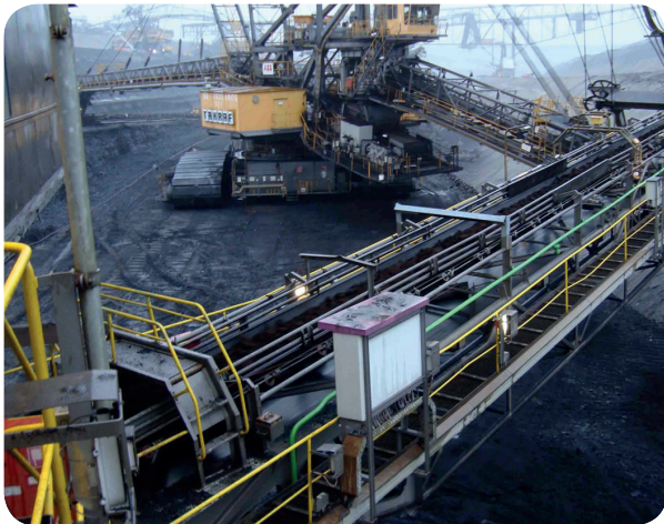
Image 2: Kontron CompactPCI Systems deliver crucial information to ensure the excavators are operated as efficiently as possible and that coal performance is optimized.
